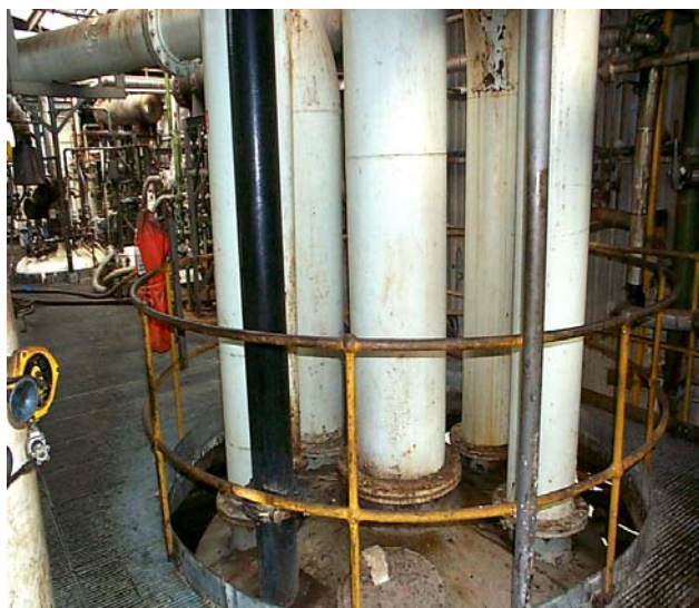
Figure 1. V7 knockout pot
