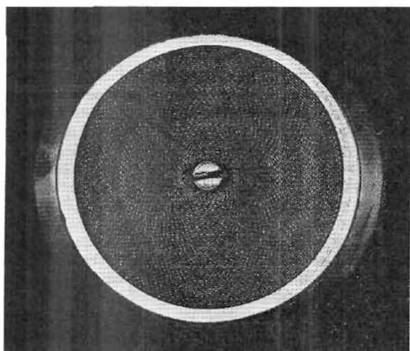
Fig. 1.—Spirally-wound crimped-ribbon arrester
