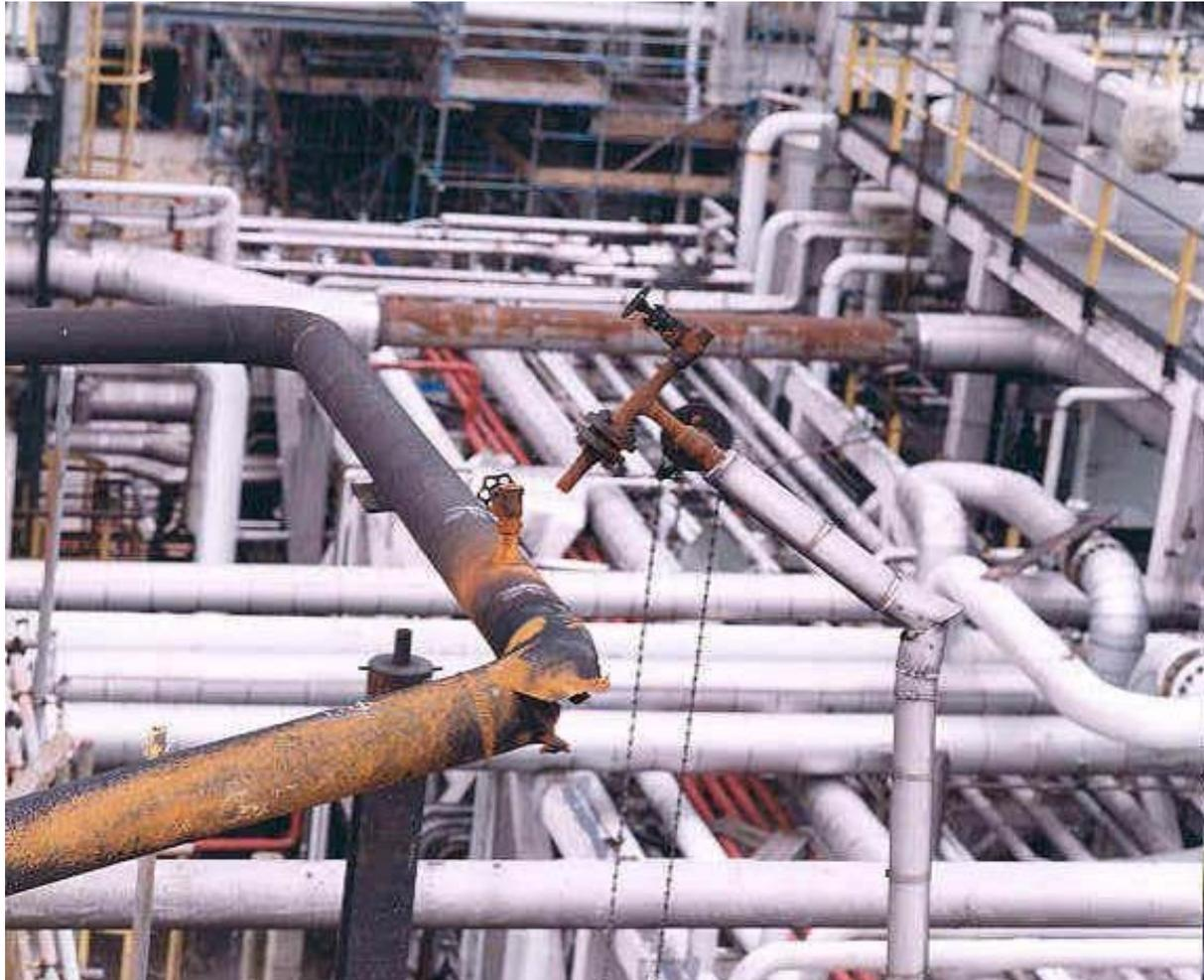
The modification had the hallmarks of a ‘quick fix’ to solve the symptoms of the immediate problem of fouling. Using an existing vent valve to connect the water into P4363 was expedient, and meant that there would have been little or no downtime required for this modification.
