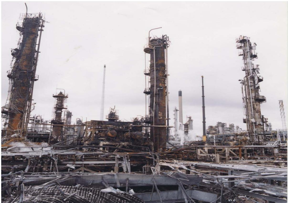
In addition buildings normally occupied on the Refinery, up to 400 metres away from the source of the explosion, were badly damaged. The contractor's canteen building suffered severe damage, had it been occupied at the time of the explosion people could have been severely injured by the flying glass. The staff canteen, the inspection services building and the toilet block suffered blast damage with windows blown in, doors and ceilings damaged and some cracking and displacement of brickwork.
