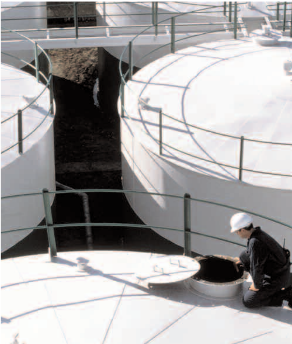
Figure 10 Maintenance worker inspecting a tank top
