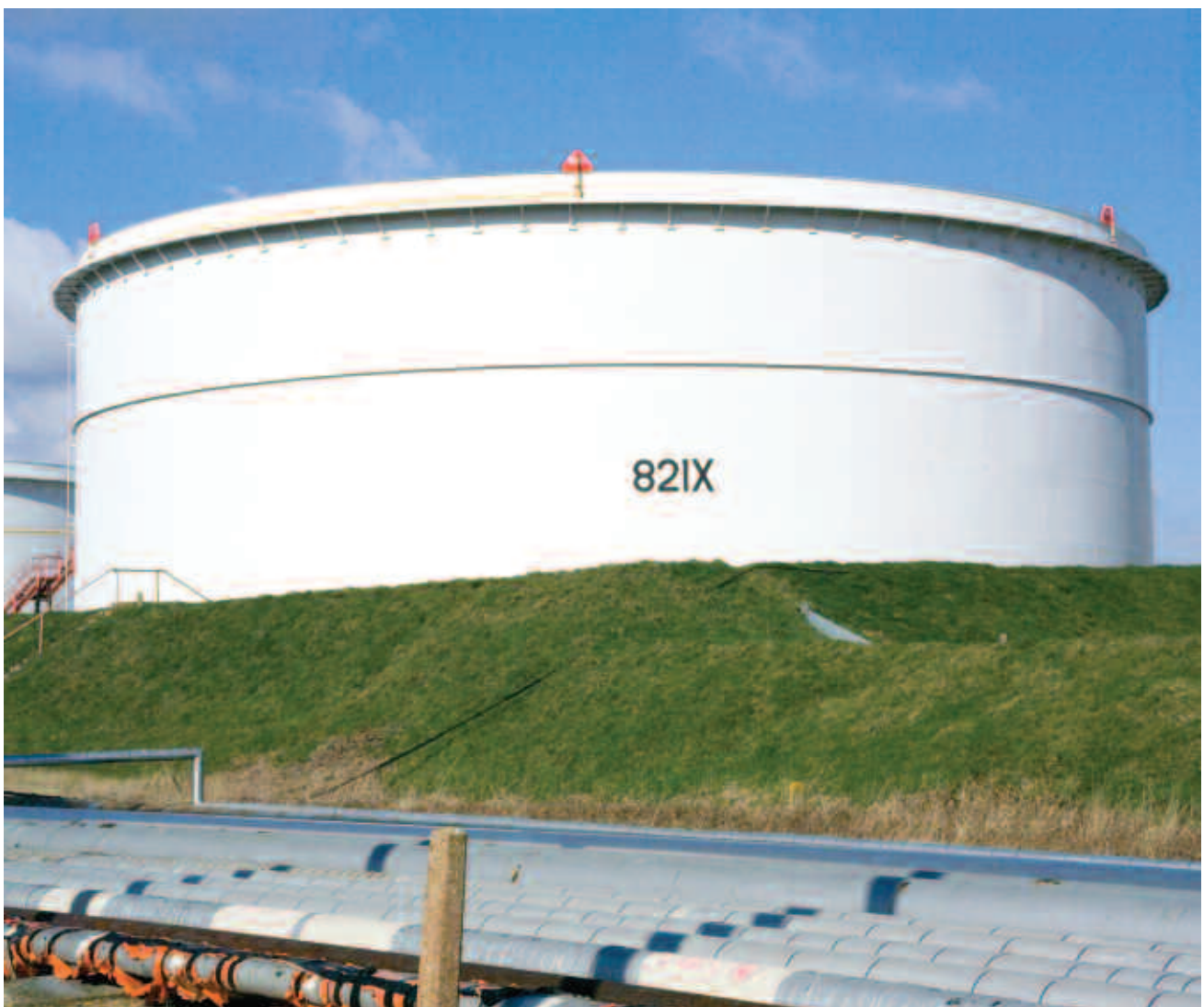
Figure 8 View of fuel tank set in earth bund
