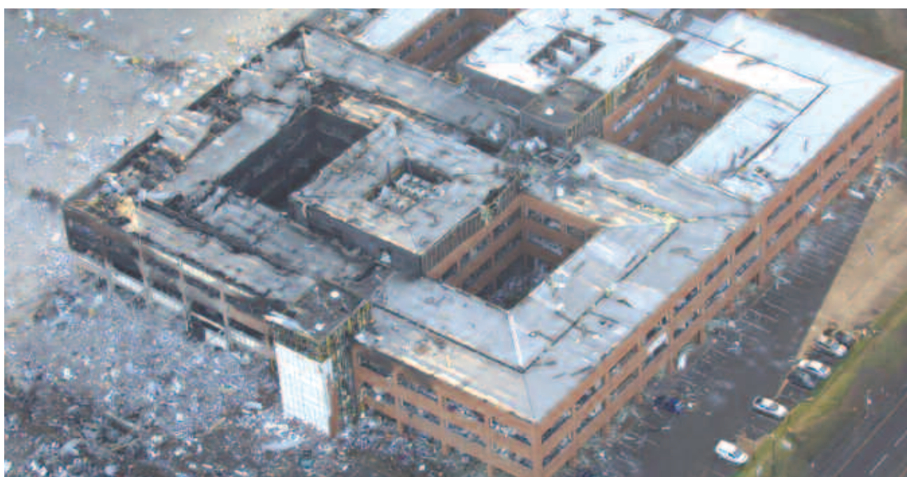
Figure 3 Damage to property on the Maylands estate adjacent to Buncefield
