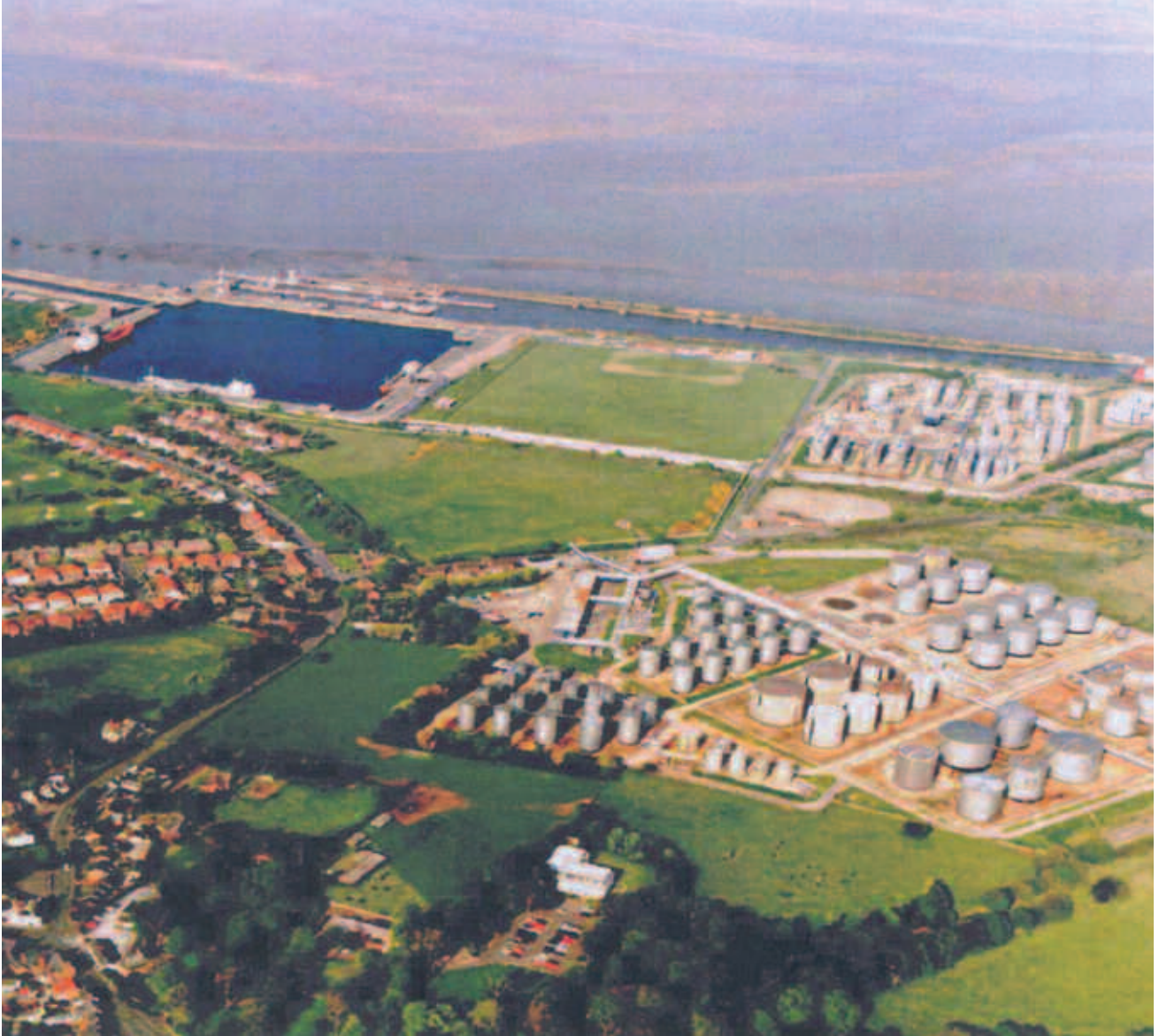
Figure 1 A general view of bulk storage facilities and ship loading facilities
