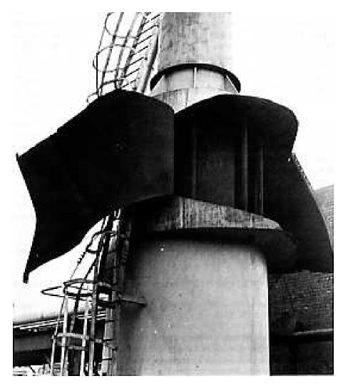
The picture shows the result of an explosion in the base of a flare stack in September 1966.
