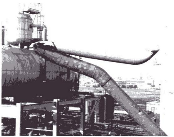
This happened in 1969 when a steam relief valve lifted and the tail pipe was not supported adequately.
