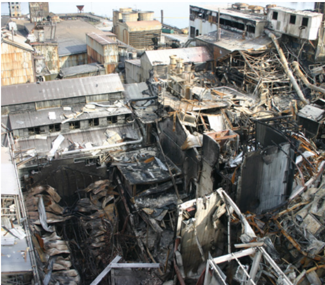
Figure 4: The extensive damage to buildings and equipment
