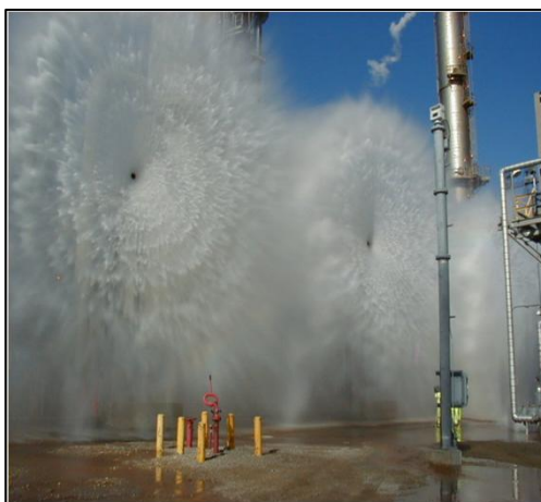
Figure 5. Water Wall Mitigation in Operation
