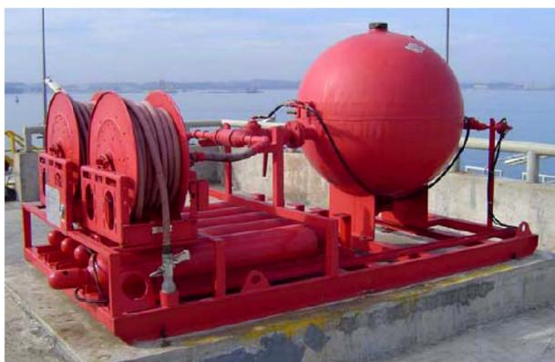
Figure 19. Example of fixed dry powder monitor
