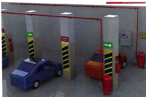
Figure 18. Example of fixed piped dry powder system
