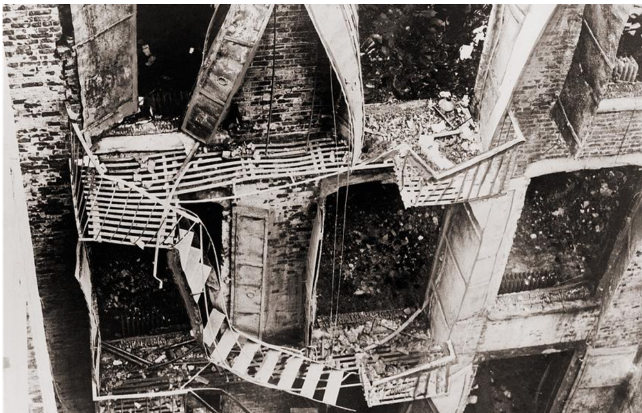
Figure 2 – The twisted remains of the fire escape and the outward opening doors at Triangle
