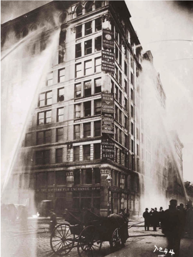
Figure 1 – The fire brigade hoses failing to reach the top floors at Triangle
