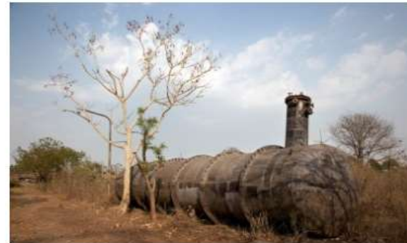
The tank that leaked the MIC gas
