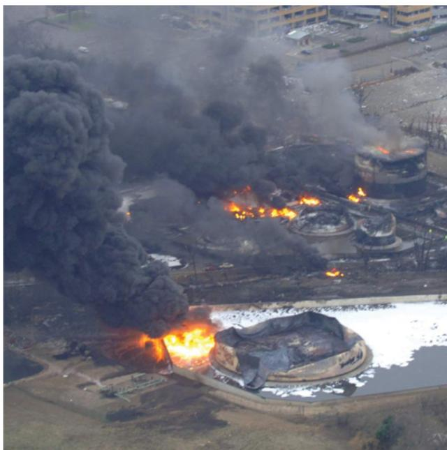
Figure 3 – Photograph taken at 15:47pm 13/12/2005 (57 hours after the explosion) (Copyright Chiltern Air Support). The photograph shows residual tank fires: Tank 912 (top right) still has a substantial inventory.
