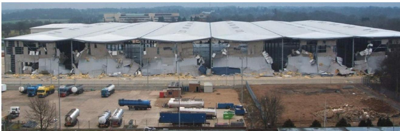
Figure 1 – Damage to a warehouse 400m from the overfilled tank (Copyright: HSE)
