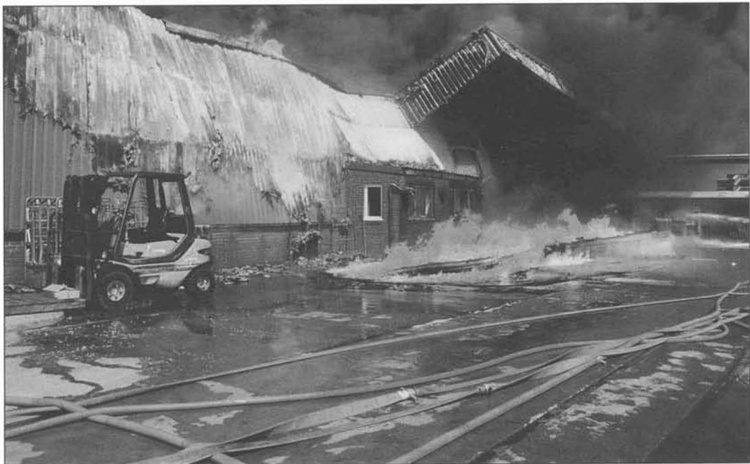
**Figure 4:** The loading bay side of the raw materials warehouse with collapsed walls and canopy, and molten flaming chemicals flowing down the ramp. Courtesy of West Yorkshire Fire Service.
