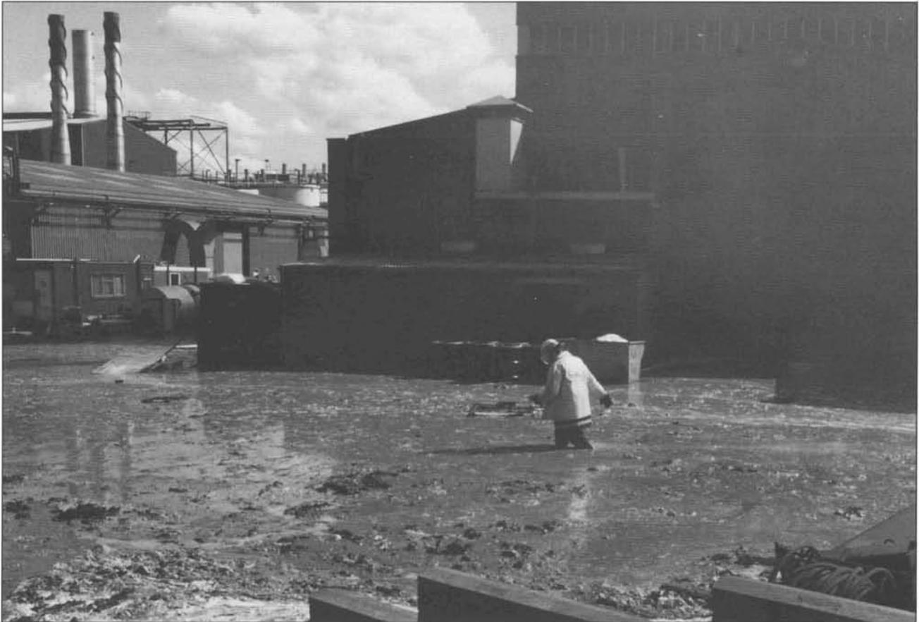
*Figure 13: Sludge-like mixture from fire-fighting water and materials from the fire affected areas which flowed downhill to the centre of the site and beyond. Courtesy of West Yorkshire Fire Service.*
