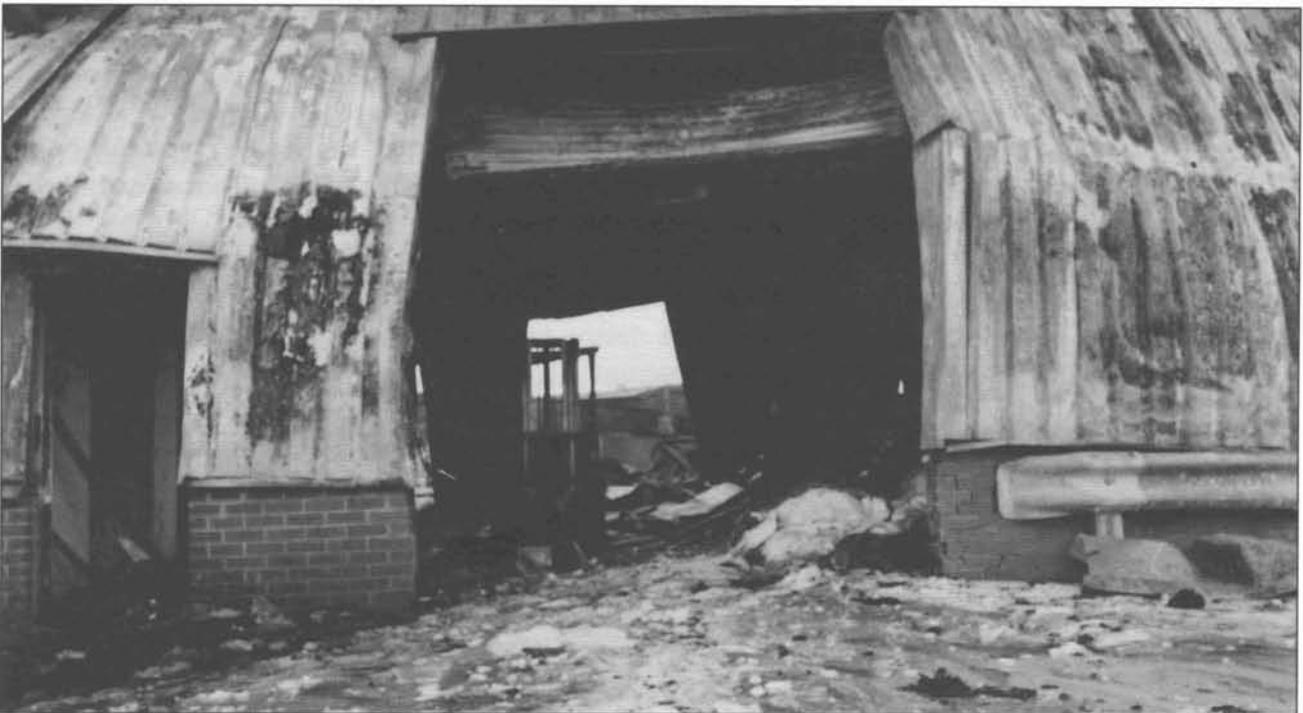
*Figure 7: Burnt out entrance to raw materials warehouse with solidified chemicals from storage inside. The door of the office where the records were kept is to the right.*
