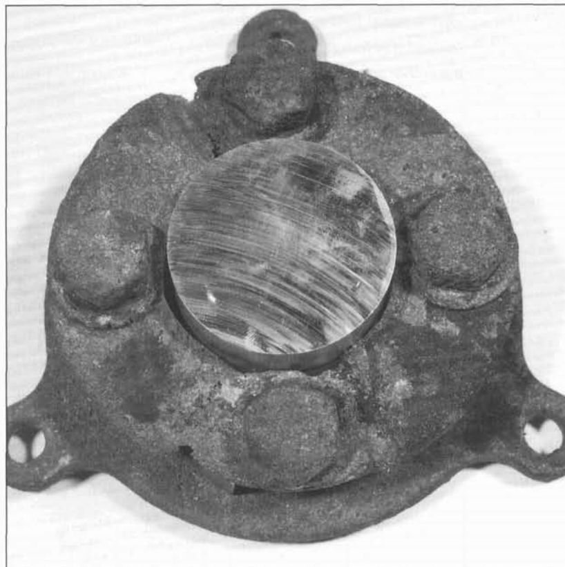
Figure 9 Photograph of corroded split flange from P251 with 50 mm brass cylinder to simulate pump discharge port
