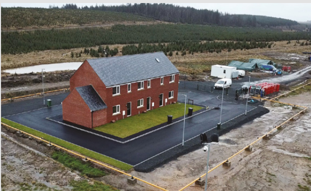
Spadeadam – Views of the H21 test houses, located at the specialist rig at DNV GL, in Spadeadam Cumbria. The houses are surrounded by a ring main that is filled with hydrogen and released in a controllable manner.
