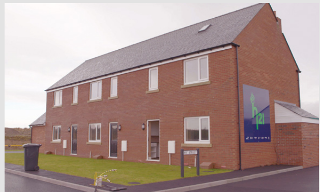
Spadeadam – Views of the H21 test houses, located at the specialist rig at DNV GL, in Spadeadam Cumbria. The houses are surrounded by a ring main that is filled with hydrogen and released in a controllable manner.
