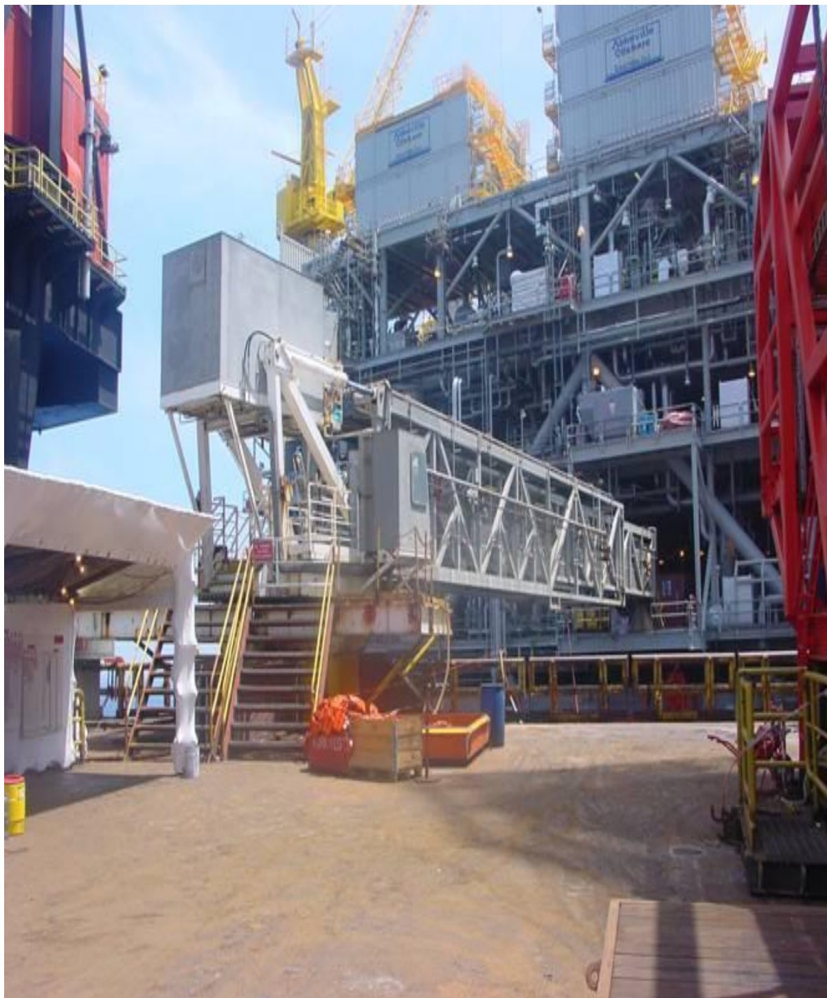
Fig (4) Bridge from the VHL to the platform
