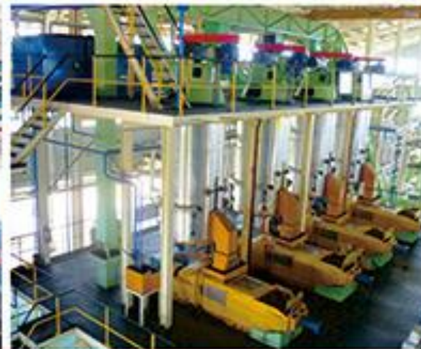
06 Digesting & Pressing station
