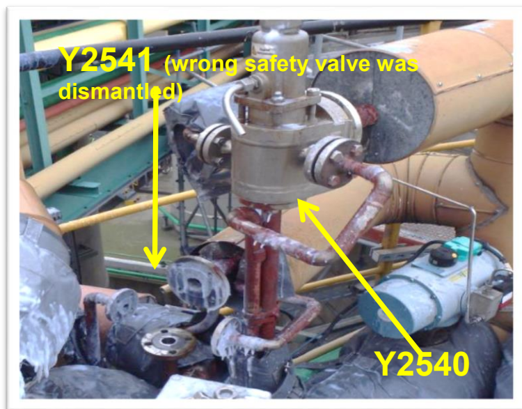
Figure 5: Leakage of sticky product
