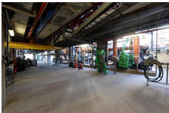
Figure 4: Pump combination (left pump is P110, right P109-120)
