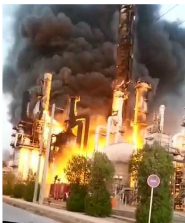
Figure 1 Paraxylene Distillation Tower (C-8001) Surrounded by Flames
