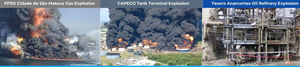
Accident was caused by a loss of condensate containment in the pump room which resulted in 9 fatalities and injuries to 26 workers. Terminal Tank fire caused by tank overfilling. It resulted in damage to 17 out of the 48 storage tanks, and environmental damage. Ignited release due to HTHA in the heat exchanger of the NHT unit. Resulting explosion and fireball caused 7 fatalities and significant asset damage.
