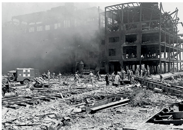
Figure 3 – Rescue workers search through debris near the Monsanto Building after the Texas City Disaster of 1947 (Courtesy of Moore Memorial Public Library, the John P. Blizetec Collection)
