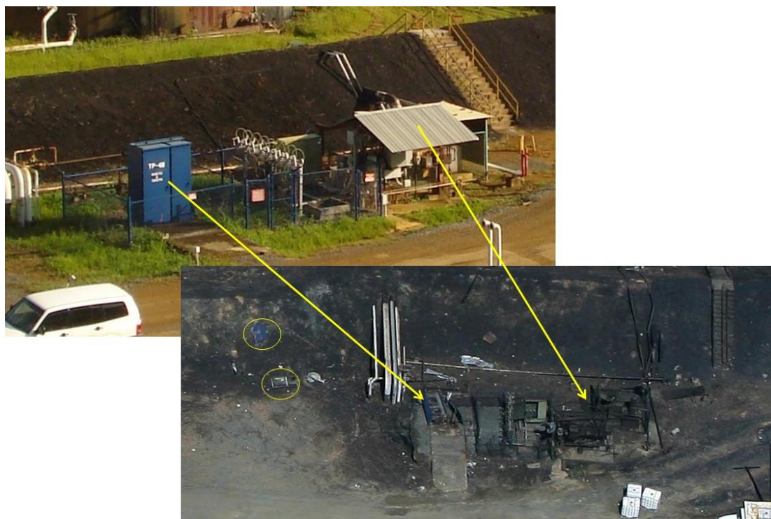
Figure 9. Secondary Ignition Location (Electrical Equipment Enclosure)
