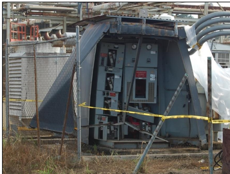
Figure 7. Ignition Source (Electrical Equipment Cabinet)
