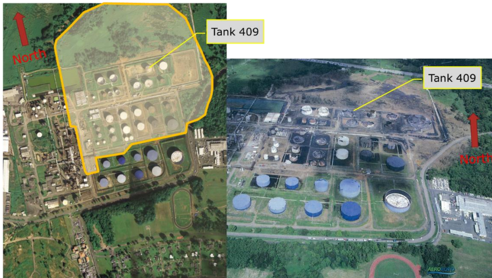
Figure 5. Flammable Cloud Overlaid on Before Photograph and Compared to After Photograph
