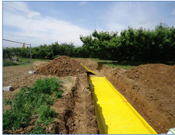
Figure 9: Example of physical protection – PE slabs
