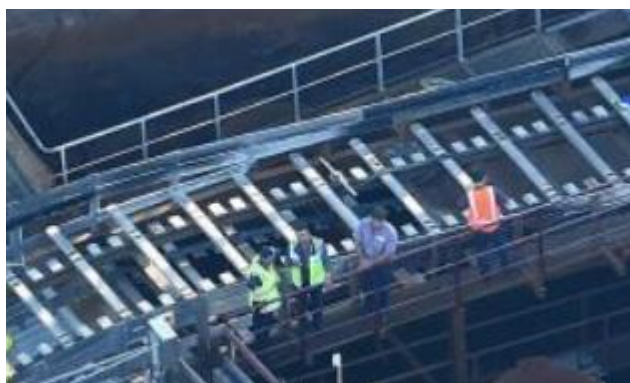
Figure 2. Aerial view of Thunder River Rapids showing the large gaps in the timber slat conveyor after the incident (Sibson, 2018).
