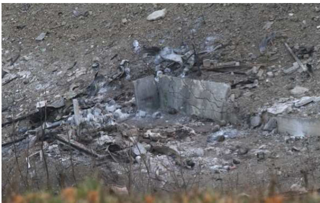
Figures 7 and 8 – Damage caused to the buildings and their protection walls
