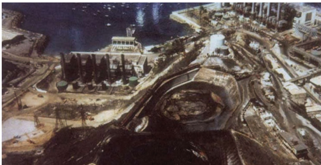
Figure 5 – Image extracted from "Incidents that Define Process Safety" shows the aftermath. Both tank 8 (foreground) and tank 9 (background) appear blackened and crumpled. Notice the steep drop-off of the dike walls and settlements underneath.
