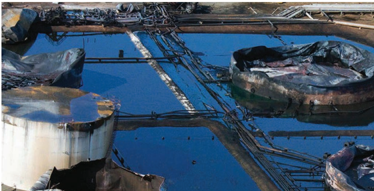
Figure 1– Firewater flooding at site
