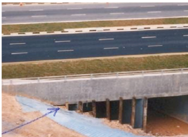
Figure 2a: Restricted access to cell 1 under carriageway
