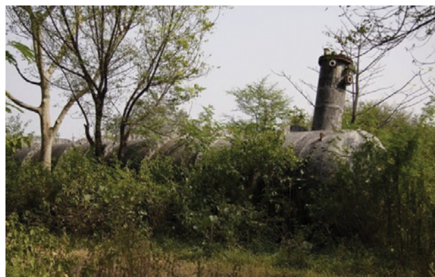
The MIC Storage tanks E610, 611 and 619 in 2014 (Julia Green www.bhopal.org )
