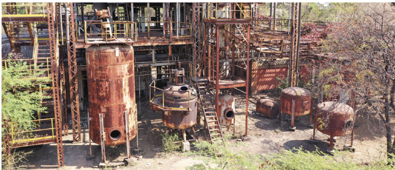
View of the abandoned Industrial gas leakage site in the Union Carbide Factory at Bhopal, Madhya Pradesh, India
