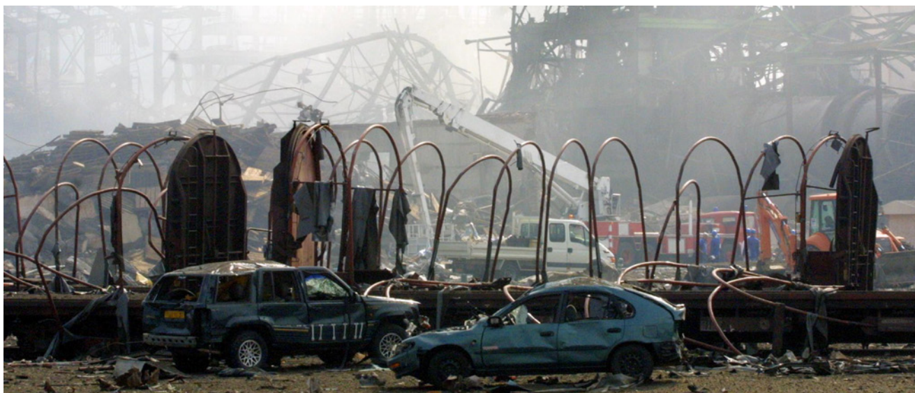
A huge explosion ripped through a chemical fertilizer plant AZF in Toulouse, France, on September 21, 2001
