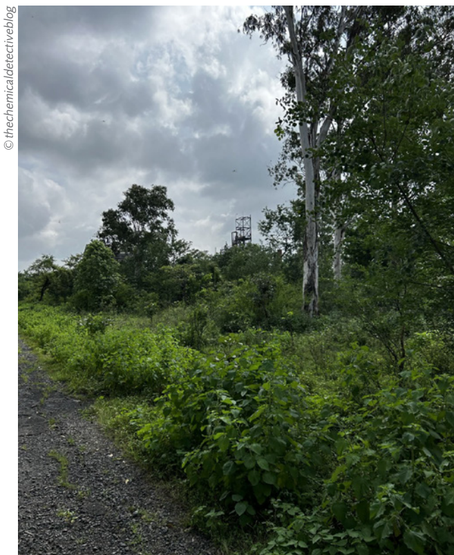
Figure 4 – Pipe bridge inside the former UCIL site in Bhopal, India, August 2023
