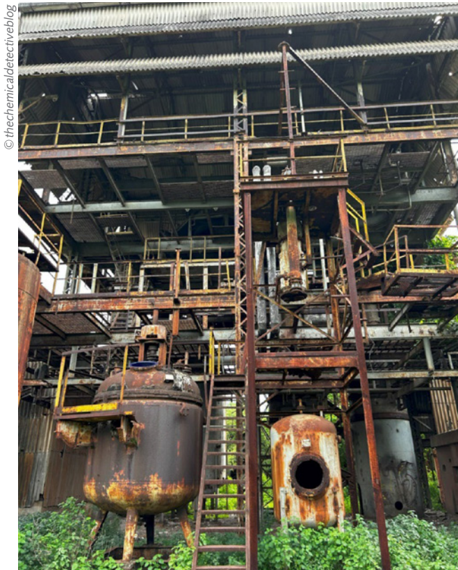
Figure 1 – Equipment at the former UCIL pesticide factory in Bhopal, India, August 2023
