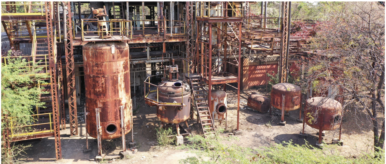
View of the abandoned Industrial gas leakage site in the Union Carbide Factory at Bhopal, Madhya Pradesh, India
