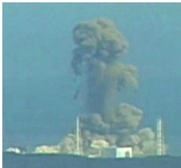
Figure 7 – Hydrogen explosion at Fukushima Daiichi 10
