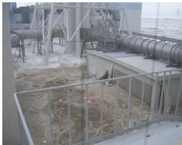
Figure 6 – Water inundation at Fukushima Daiichi 9
