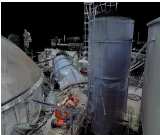
Figure 5 – The final landing position of the buffer tank at the site
