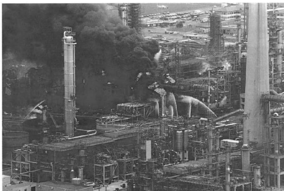
Figure 4. Fire at on plot flare knock out drum following loss of containment of flare header at Pembroke Refinery & Cracking Complex, 1994.
