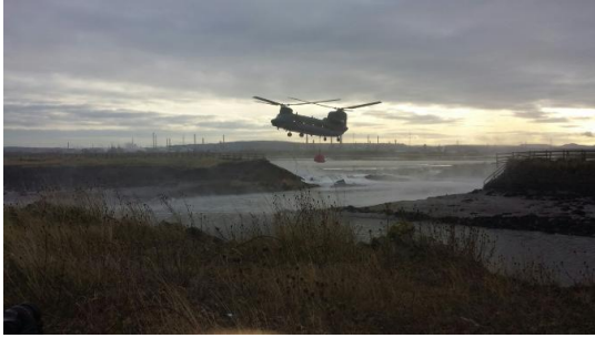
Figure 4. SABIC - Chinook helicopter dropping big bags into the breach.
