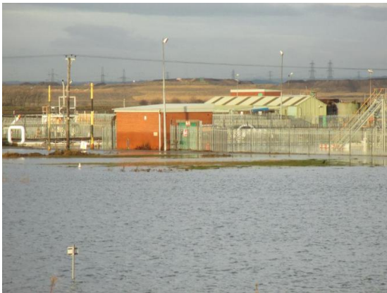
Figure 5. SABIC – note flood level mark half way up the control room wall.
