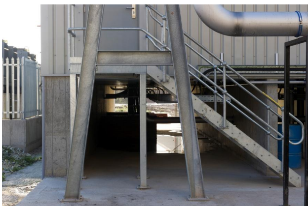
Figure 12. CEMEX – a new compressor building raised on 2m concrete plinths.
