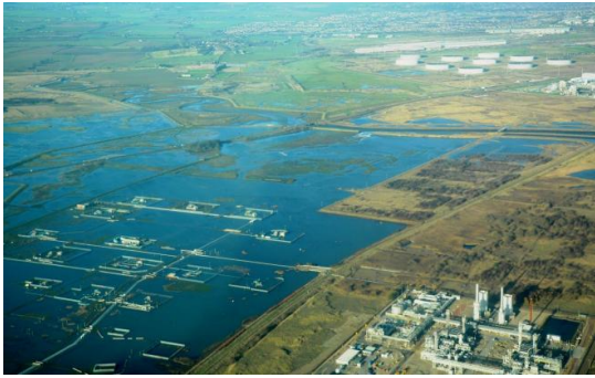
Figure 3. SABIC Brinefields and Cavities storage area showing the flood defence breach.
