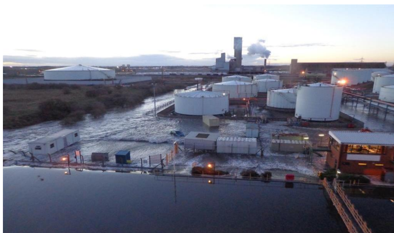
Figure 1. Inter Terminals, Riverside Terminal. Water overtopping the flood defences – as seen from a ship at the terminal.
