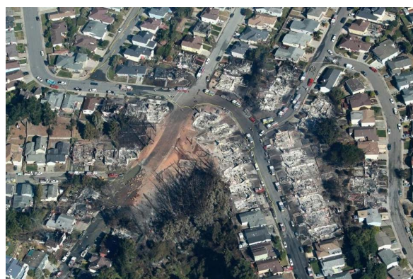
Figure 1. Gas Pipeline Incident in San Bruno, California, USA in September 2010
