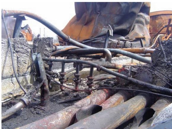
**Figure 3.** Buncefield. Catastrophic bund wall failure at pipe penetrations
