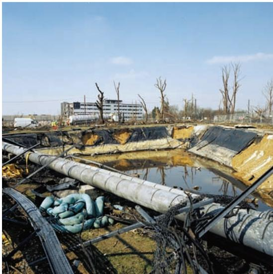
**Figure 7.** Buncefield. Damage to a lagoon liner revealing ground behind
