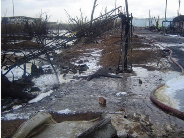
**Figure 4.** Buncefield. Contaminated fire water flowing off-site into Cherry Tree Lane
