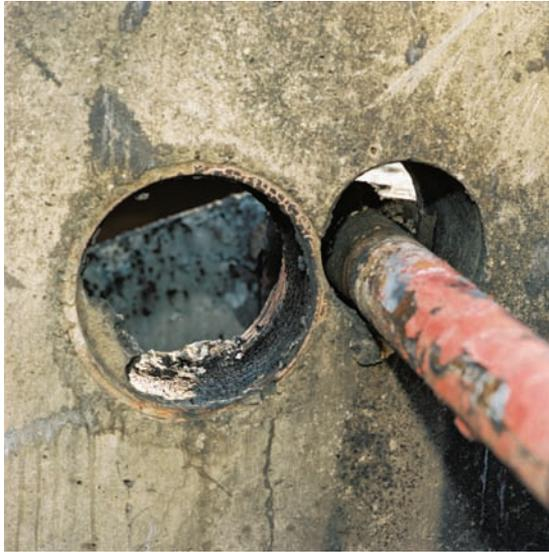
**Figure 6.** Buncefield. Loss of integrity at pipe penetrations
