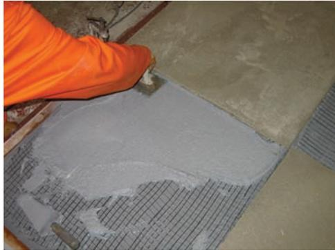
**Figure 3.** Coating Application – Butt joint
