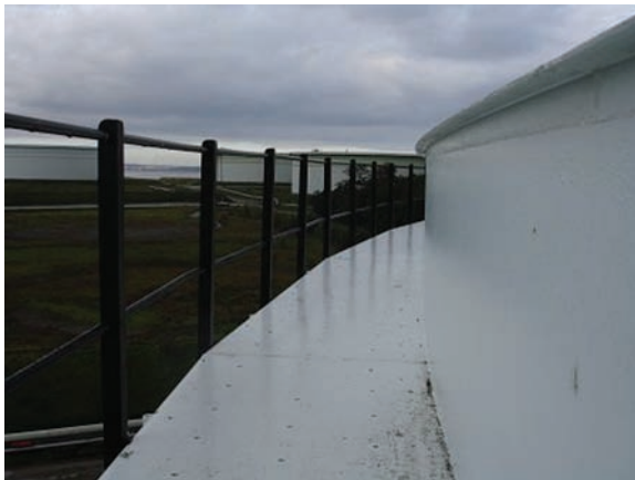
Figure 3. Top grider (walkway) in floating roof tank
