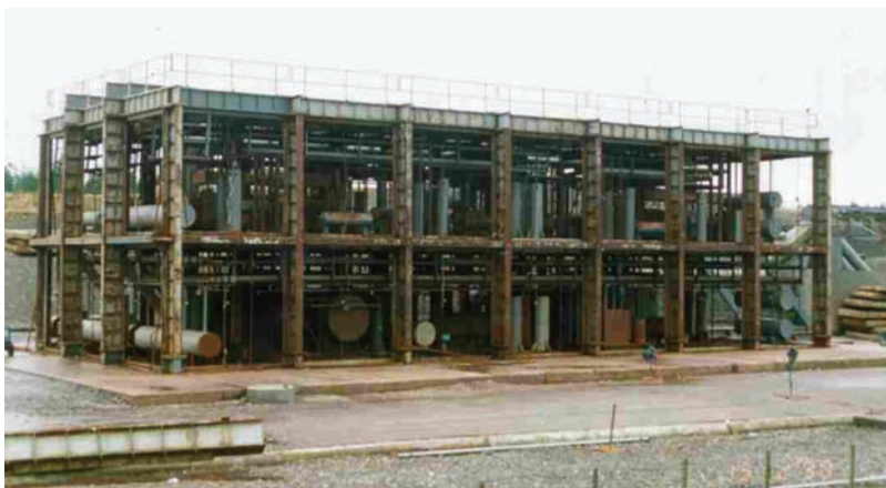
Figure 2A. A picture of the Phase 3b test rig. It measures about 28 m long, 12 m wide and 8 m high and was a large scale model of a process module on an offshore platform
